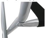
Strap ends have galvanized steel clips that are crimped, glued, and attached with screws
